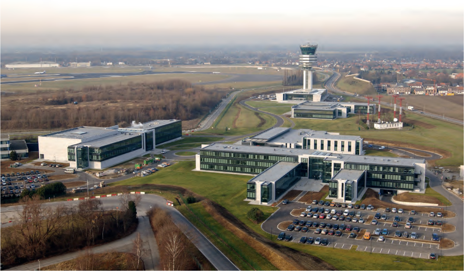
All services have been located on a brand new campus in Steenokkerzeel since April 2005.
