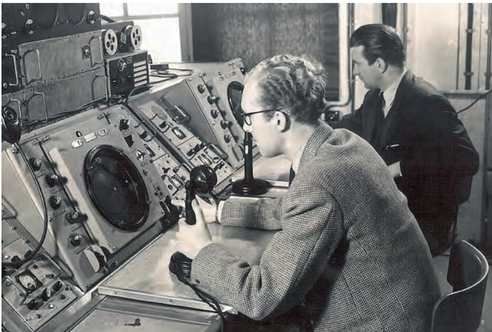
Approach controllers at work in Melsbroek, looking at the data from the direction finders
