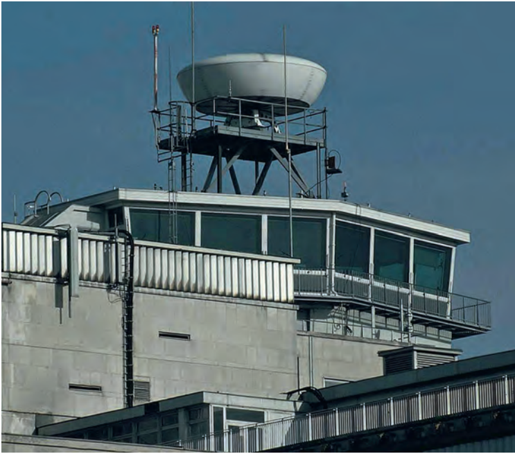
The first full, fast-turning surface movement radar is placed on the roof of the control tower of Brussels Airport.
