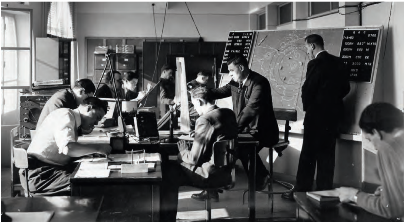
Regional air traffic control in Melsbroek, 1950
