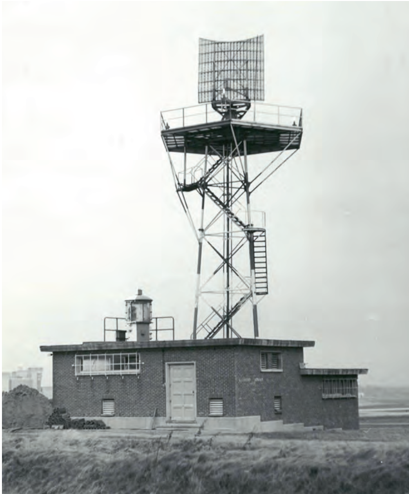
The ASR2 approach radar of 1952. It will be used for more than 20 years.
