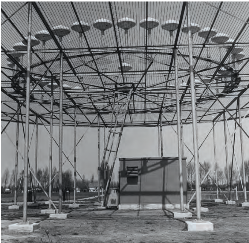
The full solid-state DVOR of Sint-Niklaas, a European first!
