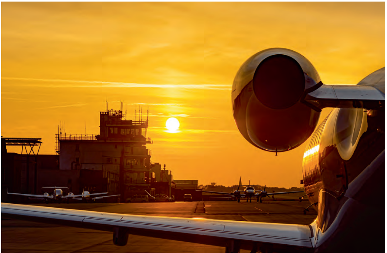
The old terminal building and the control tower at the south side of the airport
