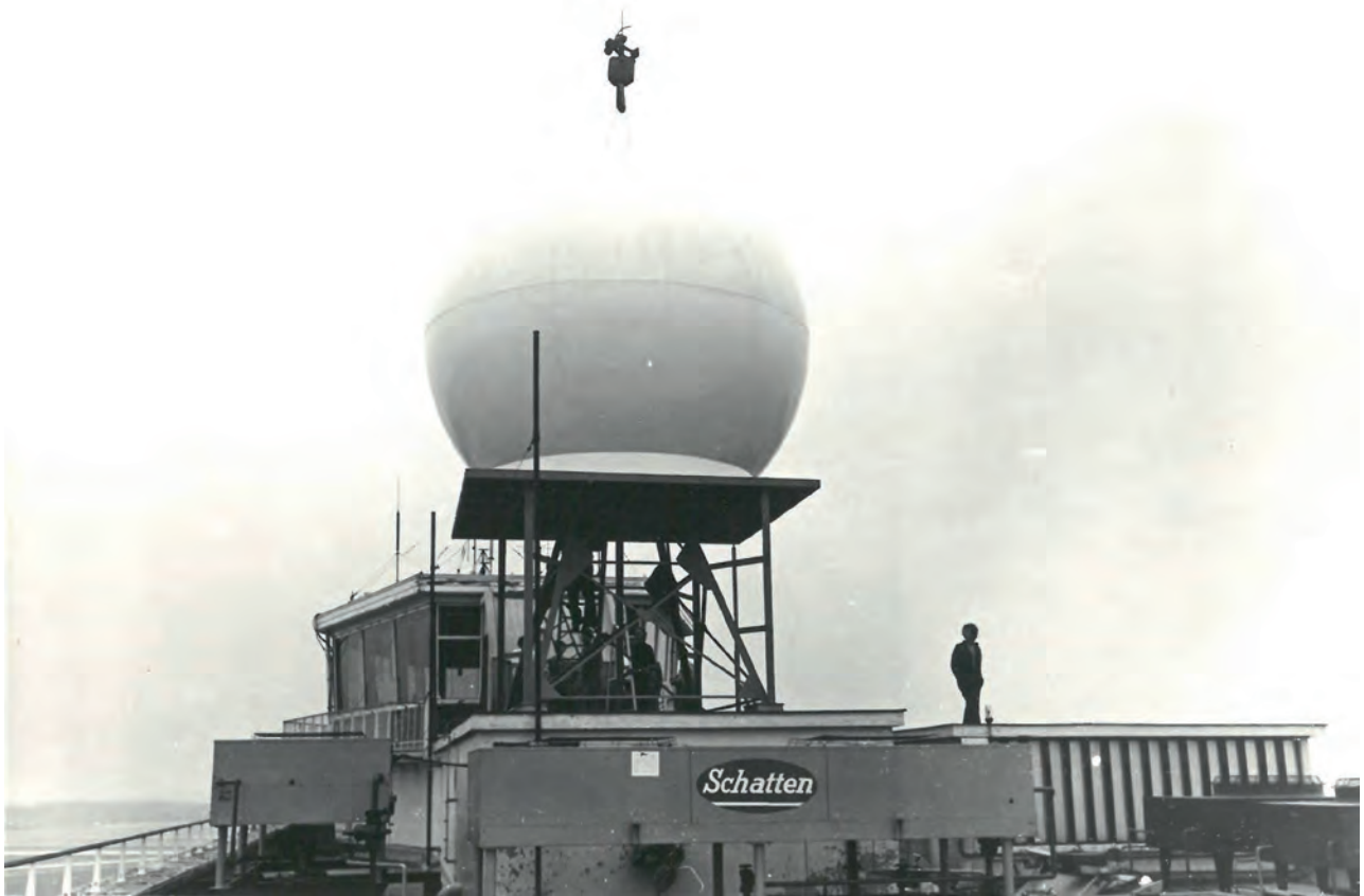
The old weather radar from 1962 is being replaced by a newer one, this time under a white radome.
