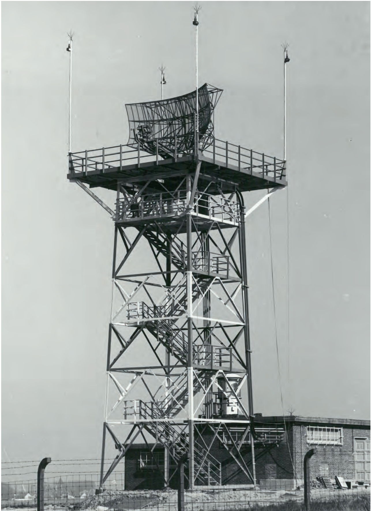
The old ASR2 is being replaced by a more efficient model: the ASR7, still a primary radar.
