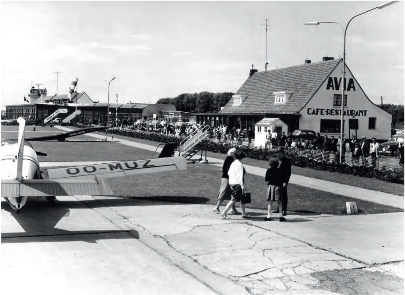
The old airport at Raversijde
